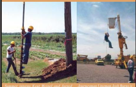
Summer interns Kent Weigel and Jarred Martens prepare the digging auger to drill a hole for a new pole, which will replace the old existing pole, providing for greater reliability.
